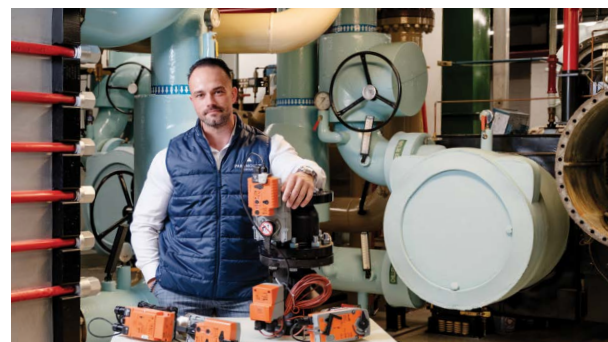
Top: 1301 Avenue of the Americas Middle and bottom: 31 West 52nd Street Opposite page: 31 West 52nd Street
